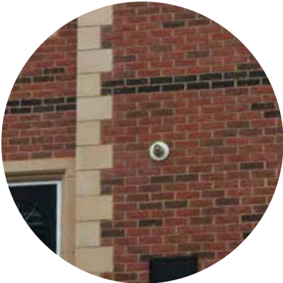
Red brick infill with sandstone trim
