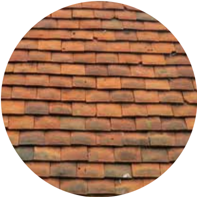
Clay hung tile on upper storeys
