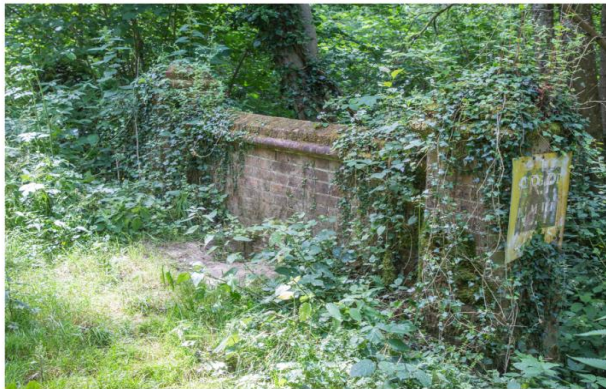
Bridge over connecting stream
