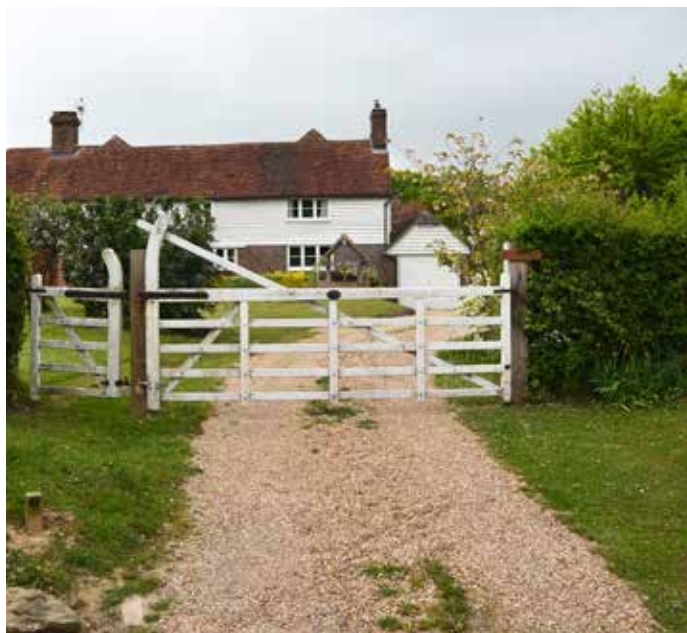
Figure 60: Use of permeable unbound gravel on a driveway
