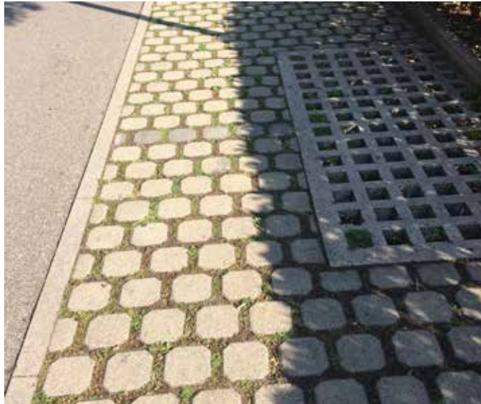
Figure 59: Examples of permeable paving (© Wikimedia Commons).
