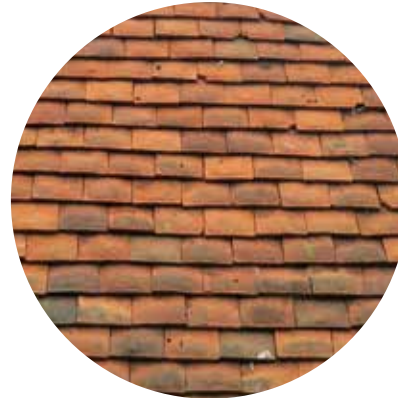
Clay hung tile on upper storeys
