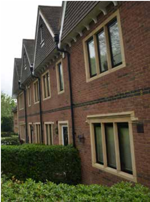
Contemporary development with brick infill, sandstone trim, and jettying gables.
