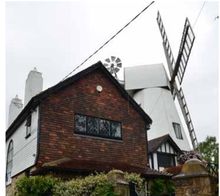
Figure 8: Grade II listed windmill on Caldbeck Hill.
