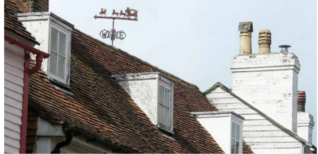
Clay plaintile roof with shed dormers and decorated weather vane.
